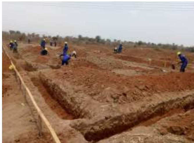
Foundation excavation in progress
