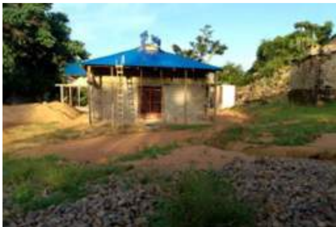
Left side of the building under rehabilitation
