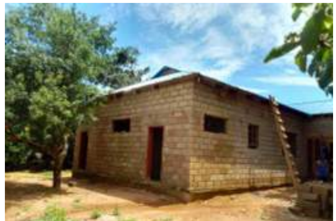
Front side of the court under rehabilitation
