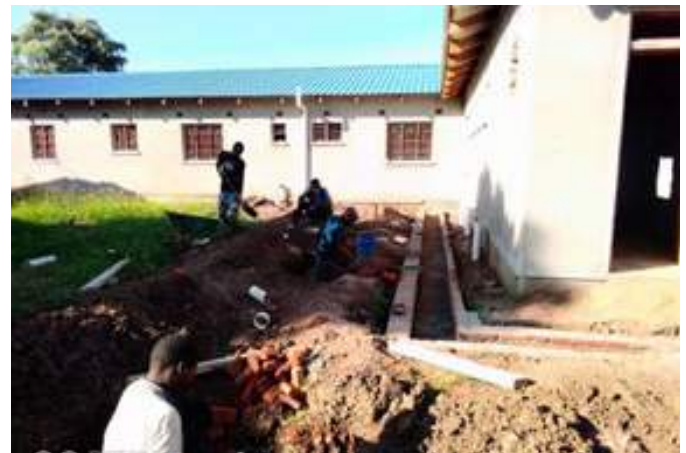
Rear side of court under rehabilitation
