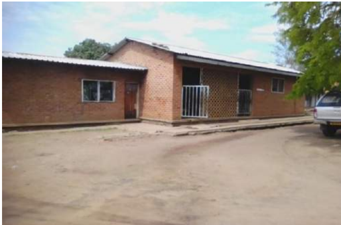
Balaka Court building before rehabilitation
