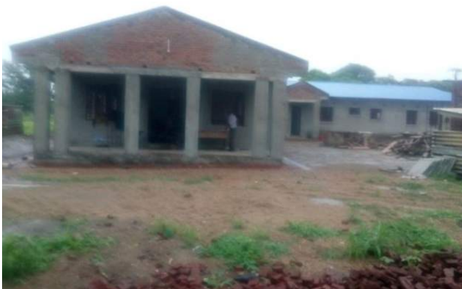
Left side building under rehabilitation
