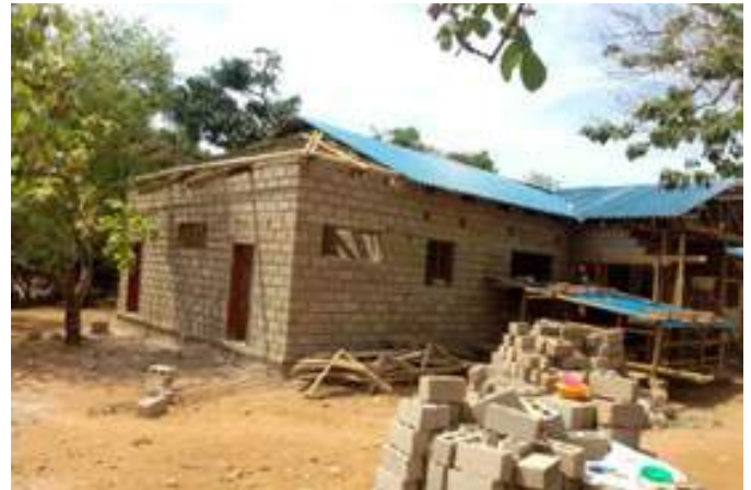
Court building under rehabilitation
