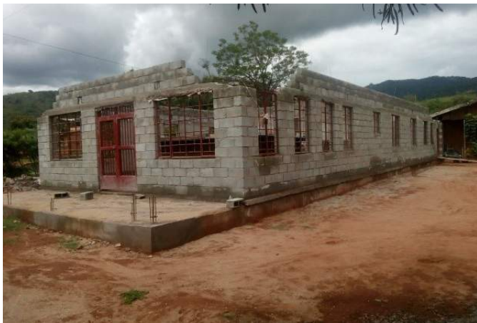
Court building under rehabilitation
