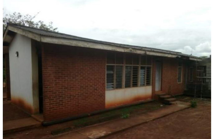
Right side building before rehabilitation
