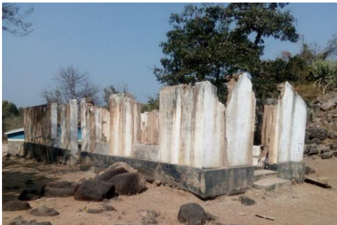
Liwonde Court building before rehabilitation
