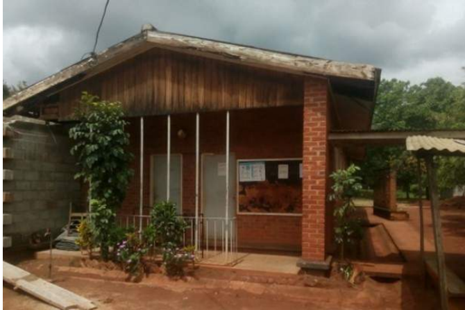
Rumphu Court building before rehabilitation
