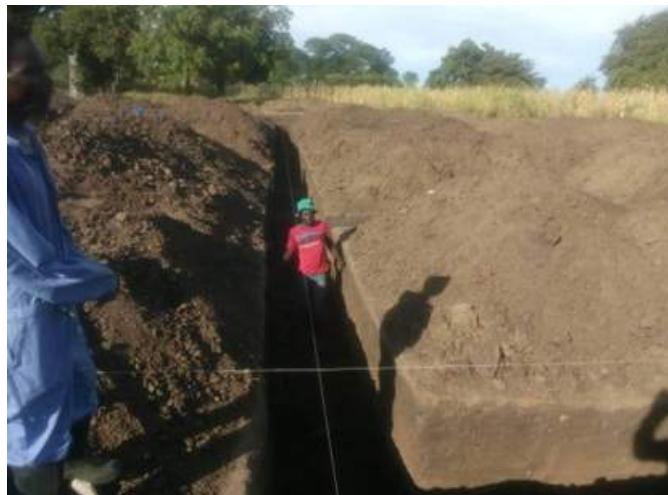
Foundation excavation in progress
