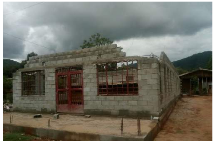
Court building under rehabilitation
