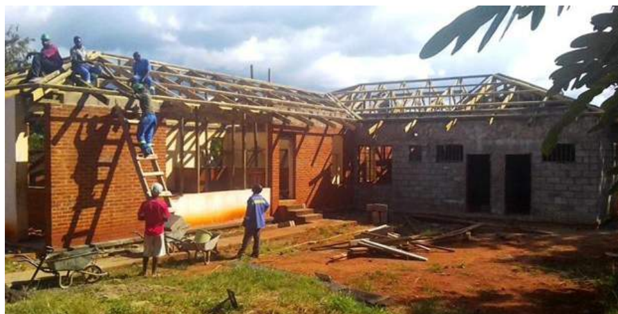
Court building under rehabilitation
