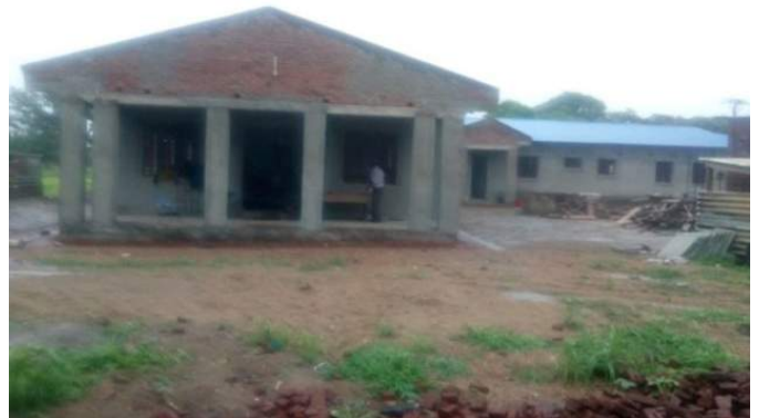
Front of Court building under rehabilitation
